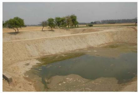
Pond Under Construction – Embankments completed but land scaping pending
