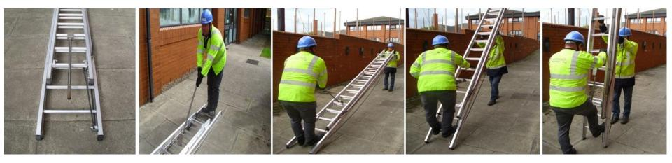
Lowering the ladder - the exact opposite of the raising procedure is followed to bring the ladder down to the ground.
