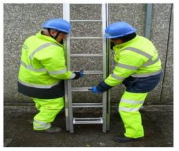
Lowering the ladder - the exact opposite of the raising procedure is followed to bring the ladder down to the ground
