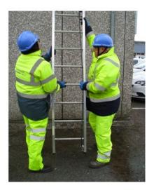
Lowering the ladder - the exact opposite of the raising procedure is followed to bring the ladder down to the ground
