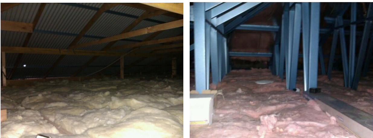
Figure 13 Examples of ceiling insulation rated as average
