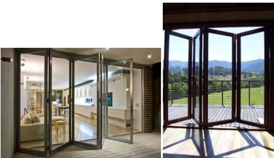
Figure 37 Examples of typical bi-fold doors showing the gaps between each door
