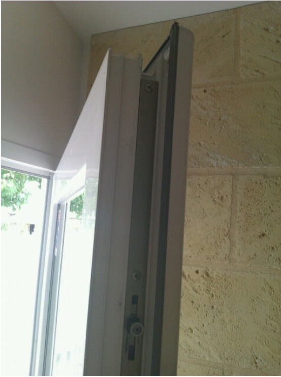
Figure 27 Examples of seals on uPVC windows and door frames
